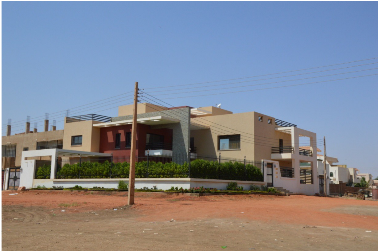
Figure 3. A new-build house in the Kafouri neighbourhood, where sales prices for villas can reach into the millions of dollars
